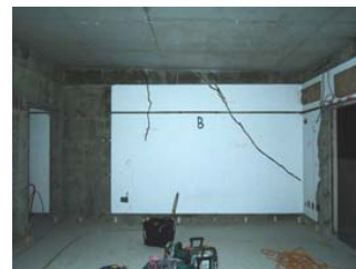
ひび割れ補修
